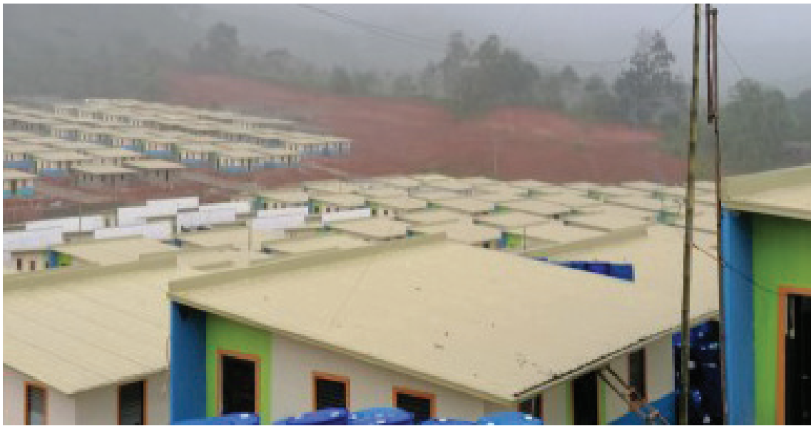
MARAWI REHAB. A view of the permanent shelter project site in Marawi City in this undated photo. President Ferdinand R. Marcos Jr. on Nov. 28, 2024 created the Office of the Presidential Adviser for Marawi Rehabilitation and Development (OPAMRD) to oversee and ensure "efficient, effective, and timely" implementation of the programs, activities, and projects under the Bangon Marawi Comprehensive Rehabilitation and Recovery Program. (Photo courtesy of DHSUD)
