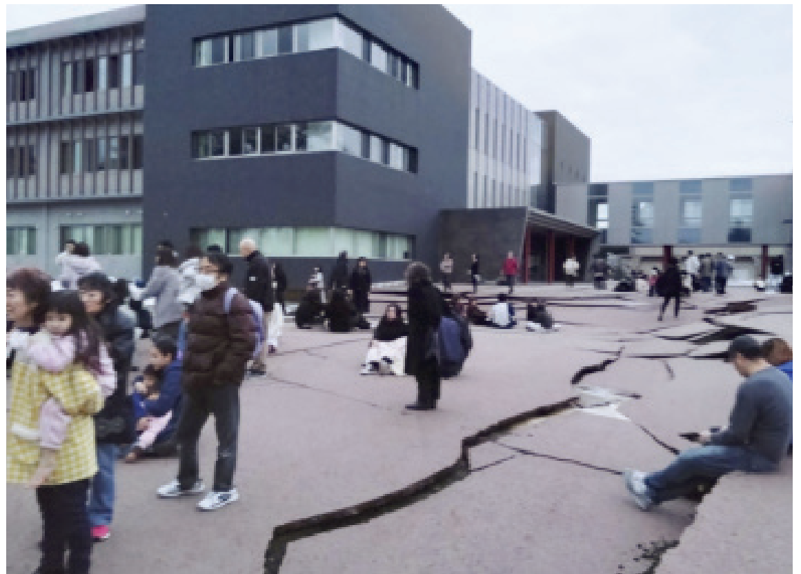
AFTERMATH. Large cracks are seen on the ground in Wajima, Ishikawa Prefecture, on Monday (Jan. 1, 2024), after a strong earthquake rocked a wide area on the Sea of Japan coast in central Japan. The Philippine Embassy in Tokyo said assistance is ready for affected Filipinos. (Kyodo photo)
