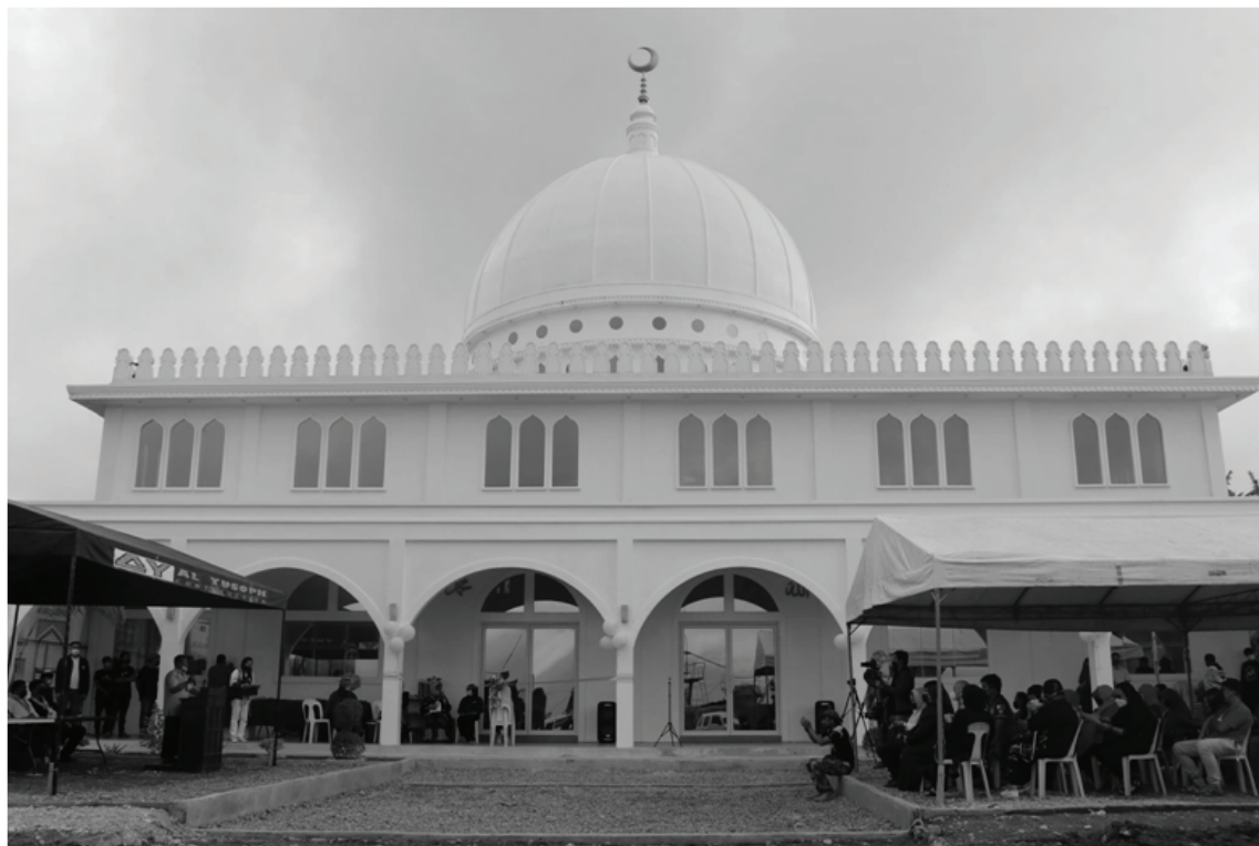
Through donations from private housing developers in the country, TFBM managed to restore, so far, five religious sites inside the most affected area. Among these is the White Mosque located in Brgy. Lumbaca Madaya.
